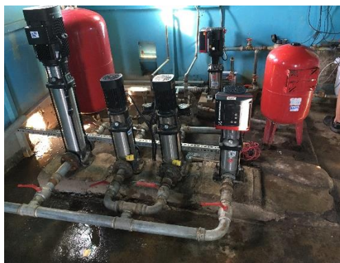
Station existante de Koteyo
